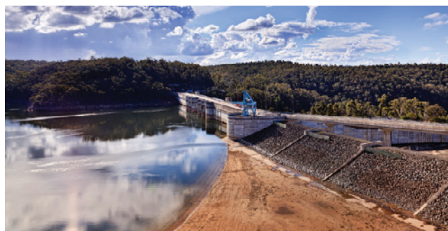
Warragamba Dam, New South Wales
