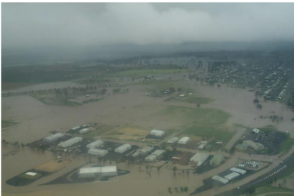
Figure 13. Aerial image of the 2004 flood for Narrabri of the Francis Street Industrial Estate 3
