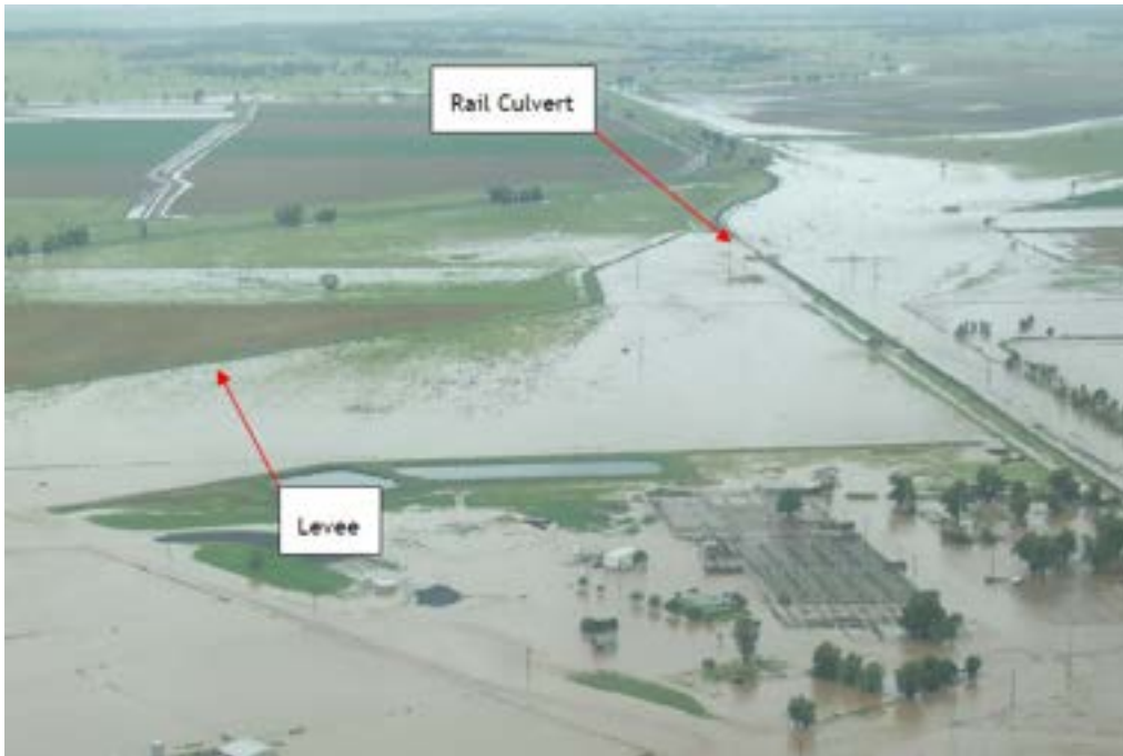
Figure 12. Aerial image of the 2004 flood for Narrabri (within Horse Arm Creek) 7
