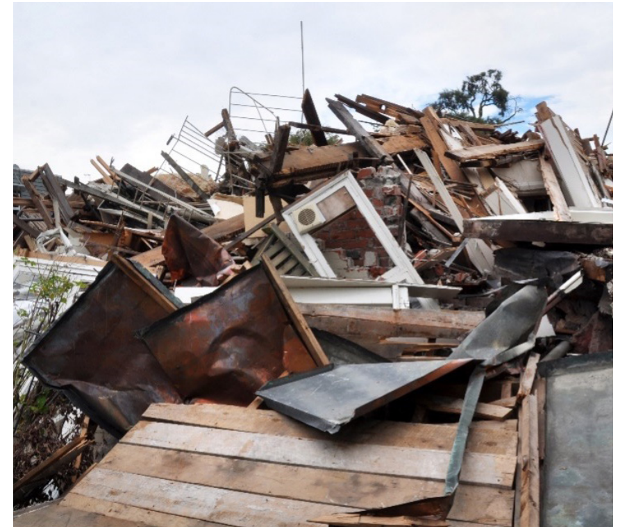
Christchurch (NZ) – Remains of a building damaged from the 2011 earthquake 18
