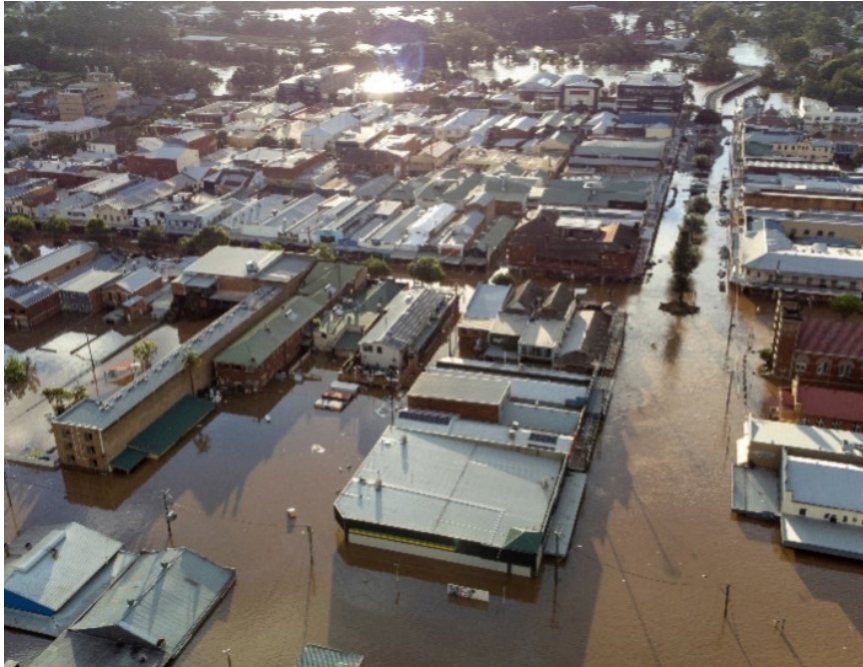
Lismore (NSW) during 2022 Floods 16
