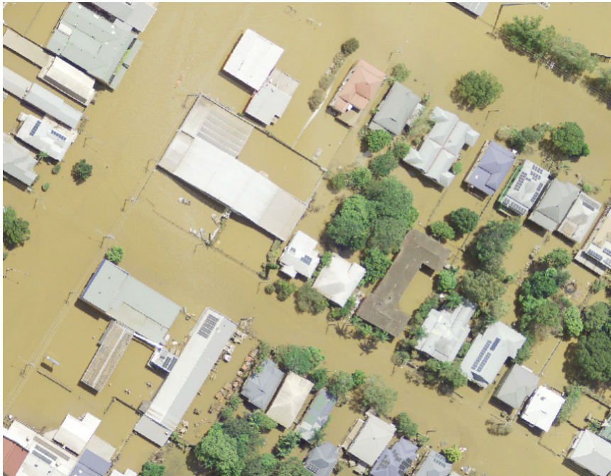
Lismore (NSW) – March 2022 flooding 3
